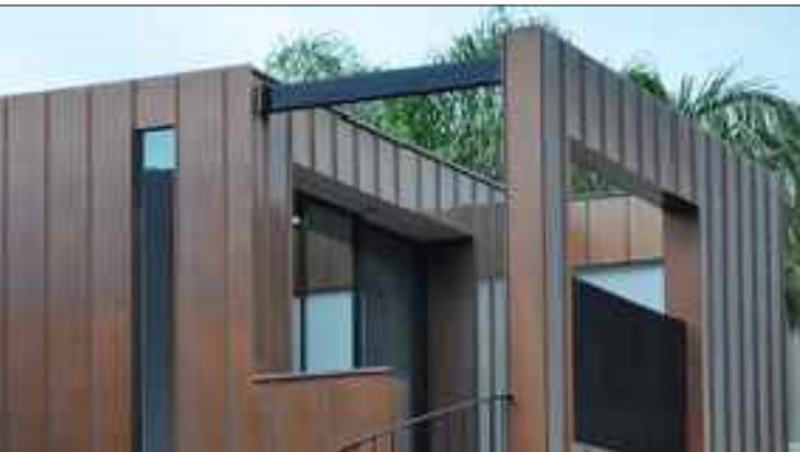
aluminum cladding aged copper standing seam aluminum cladding or similar approved cladding
