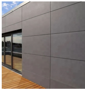
05. PPC Aluminium cladding system, warm mid grey colour or similar approved
